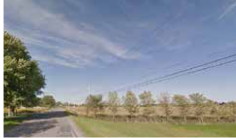
Photo : Google Street View
