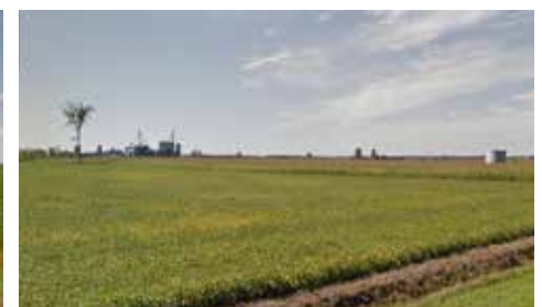
Photo : Google Street View
